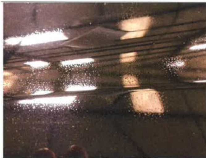
Close up of hood showing blistering
